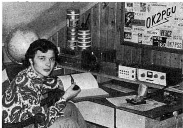
Rosti, OK2PGU, runs this largely home-built station on 1.8MHz. He uses a 125ft vertical transmitting antenna and a Beverage for receiving. (Photo: W1BB)
